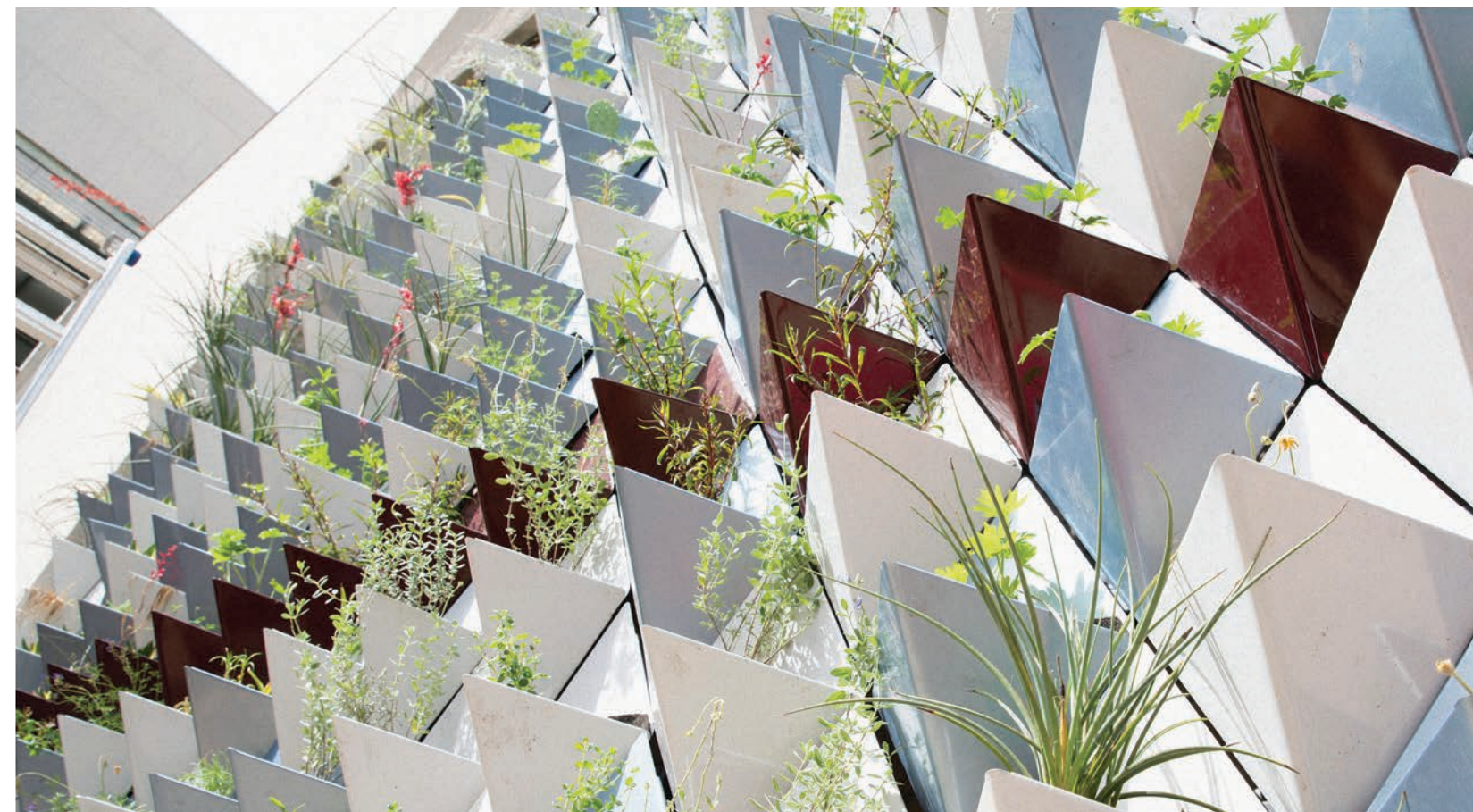
The Langford Living Wall, a unique structure made of 300 planters made from auto industry waste, sits on the Texas A&M campus on the side of Langford Architecture Center Building B.
